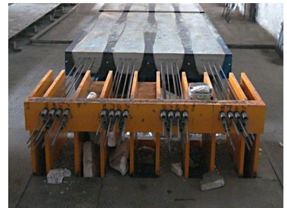
Post-tensioned cables
